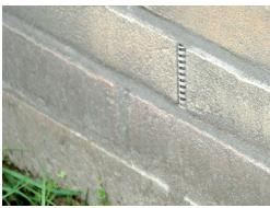
The Weephole Cover is mounted correctly when the front is equal with the cavity front. The grill will then be firmly secured in the cavity.
