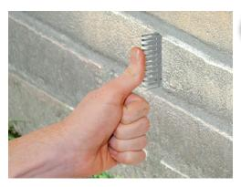
Push the Weephole Cover further into the weep hole.
